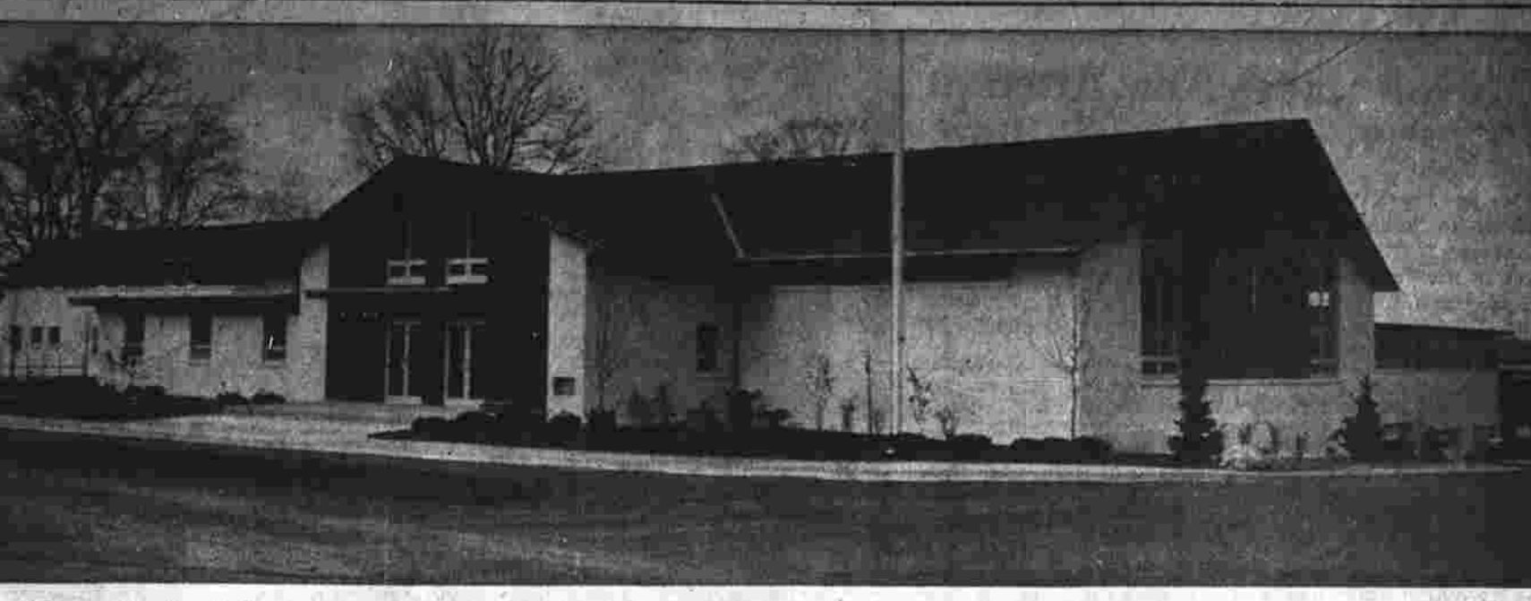
The architectural theme is rural contemporary—off-white brick block and tobacco shed wood paneling for a subdued effect.
