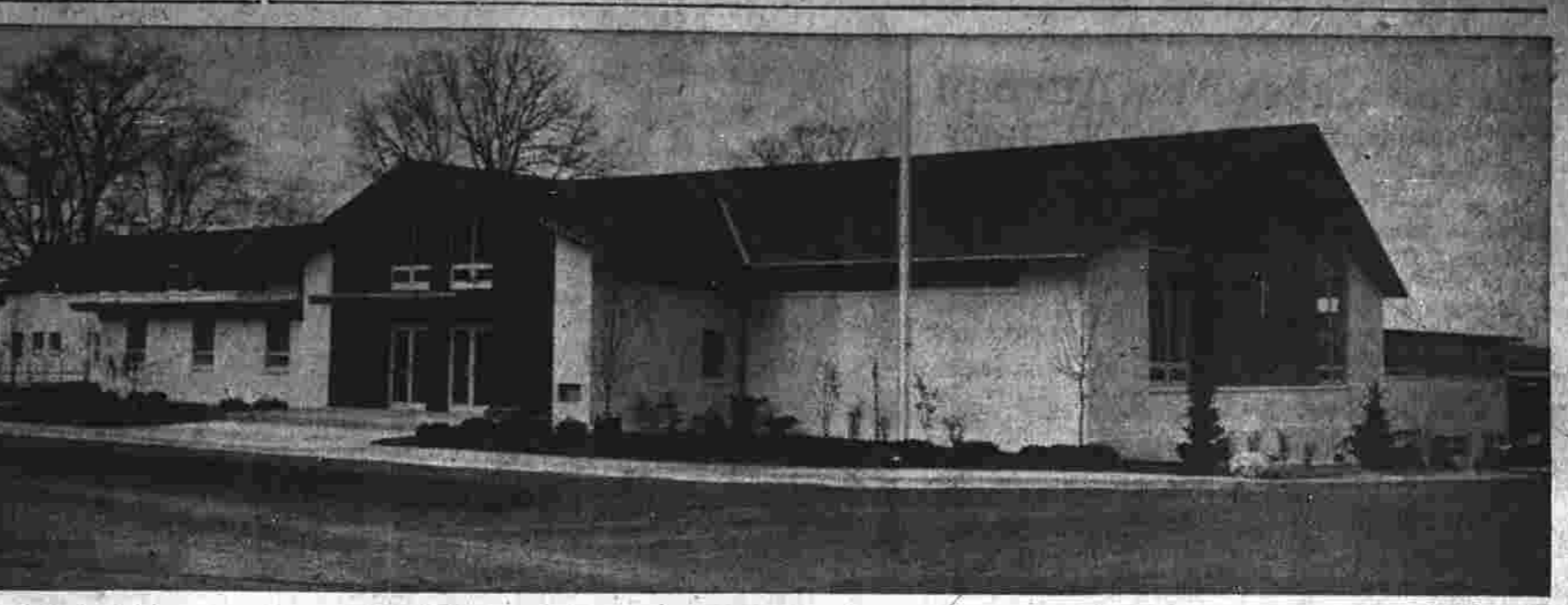
The architectural theme is rural contemporary—off-white brick block and tobacco shed wood paneling for a subdued effect.
